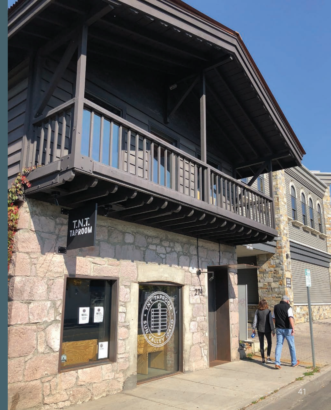
The Dynamite Shed (1880) - This building was the original storage location for explosives sold by the Gillette & Evans hardware store on Main Street which was the chief supplier of mining supplies during the mining and smelting boom. The second story was added in 1995. Photo Credit: City of Ketchum 2020
