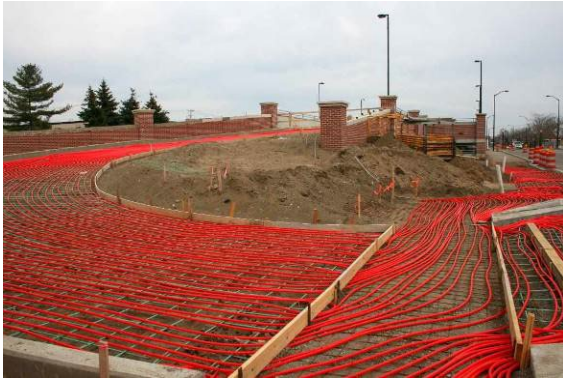
Example of the snowmelt tubing under pavers or in concrete slabs.
