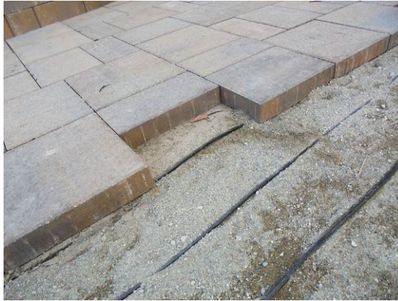
Pavers with radiant snowmelt system integrated.
