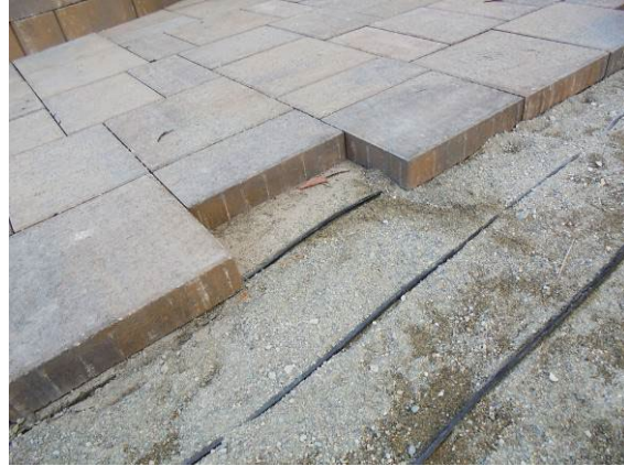
Example of the snowmelt tubing under pavers or in concrete slabs.
