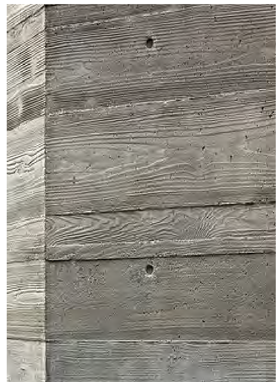
BOARD-FORMED CONCRETE - cast-in-place and stained.
