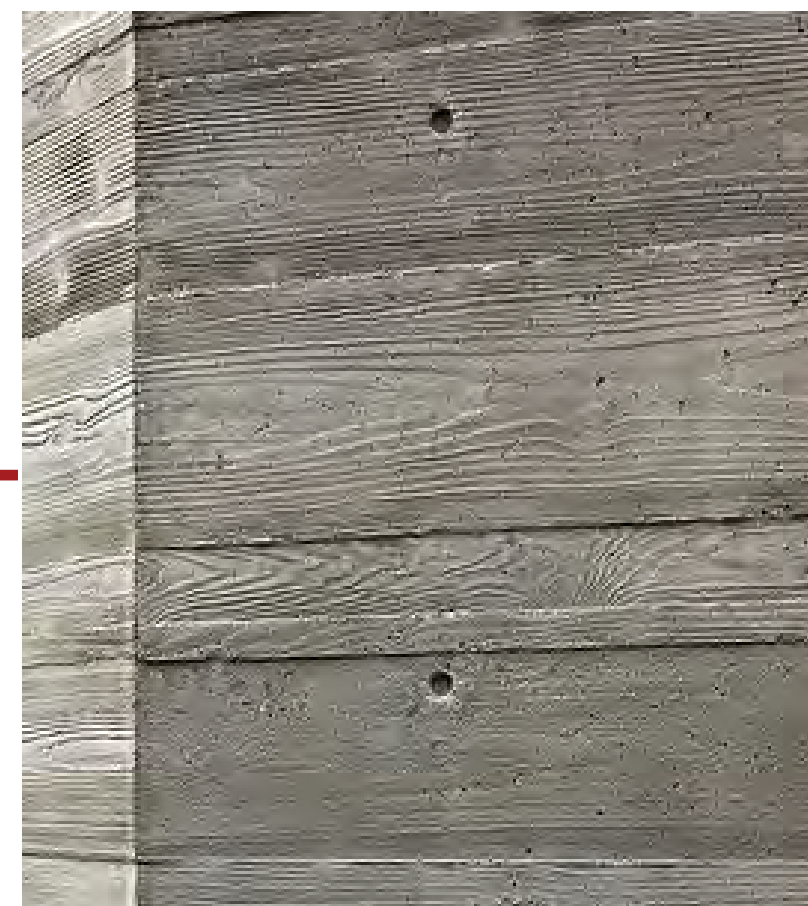
BOARD-FORMED CONCRETE - cast-in-place and stained.
