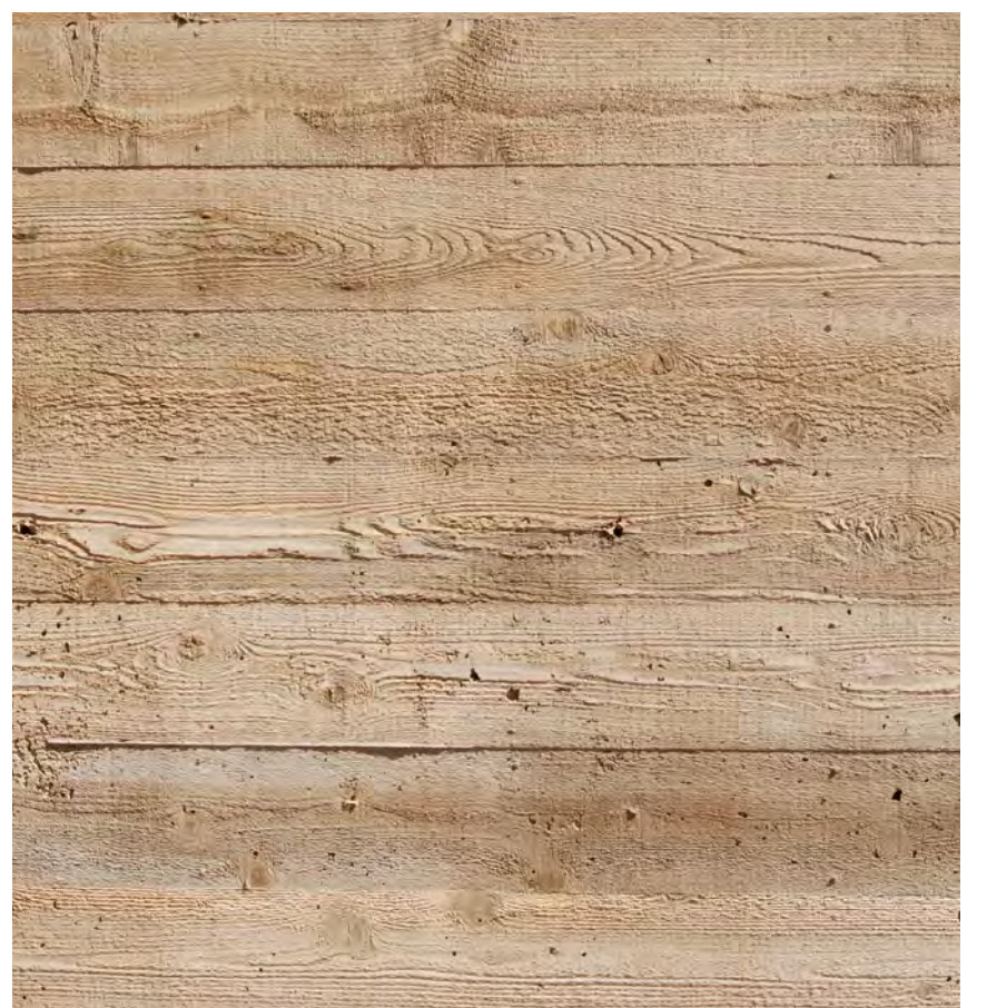
BOARD-FORMED CONCRETE - cast-in-place and stained.
