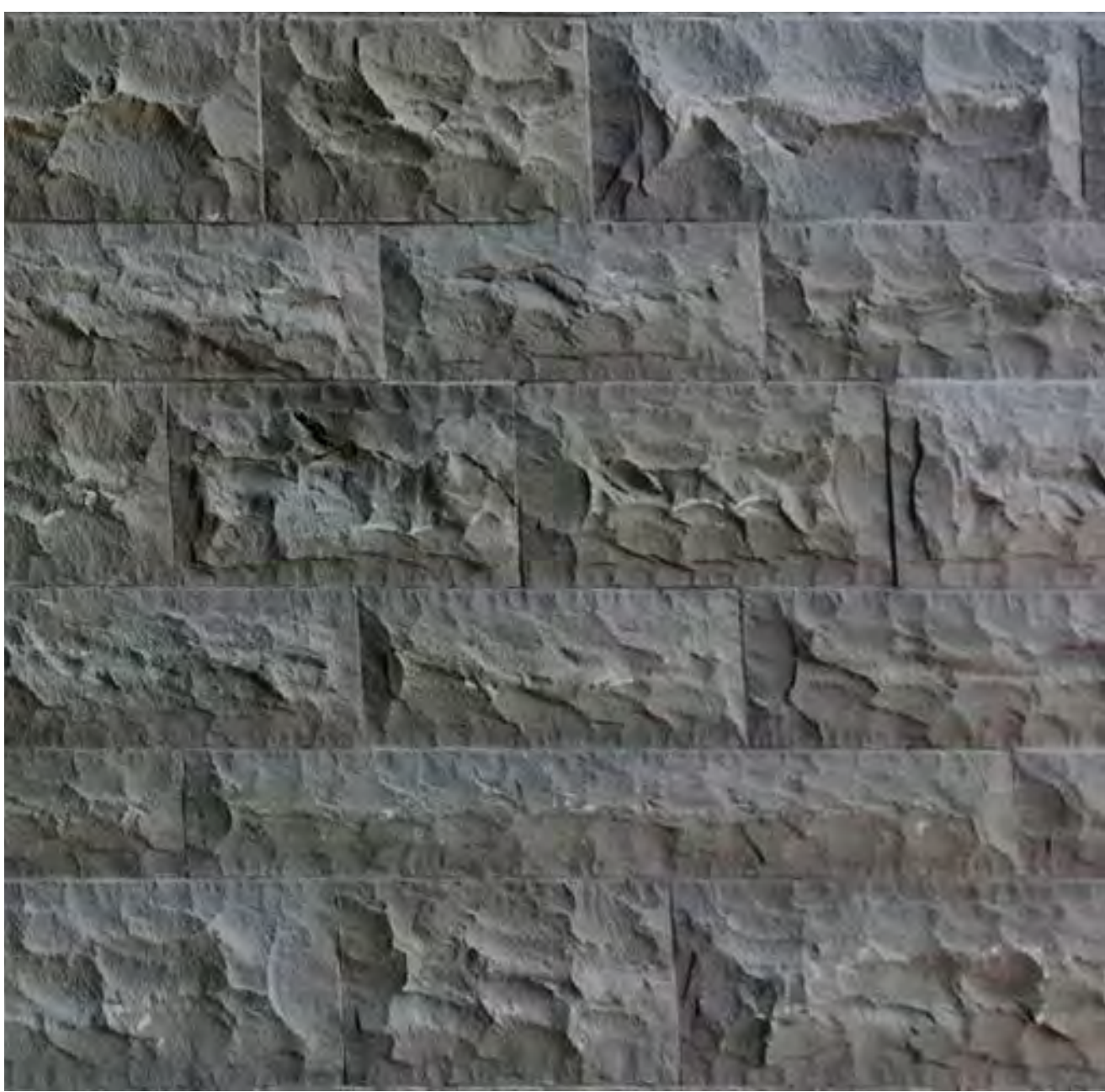
STONE VENEER - 4" thick natural stone with varying height. Dry-stack lay-up with stainless steel masonry anchor system.
