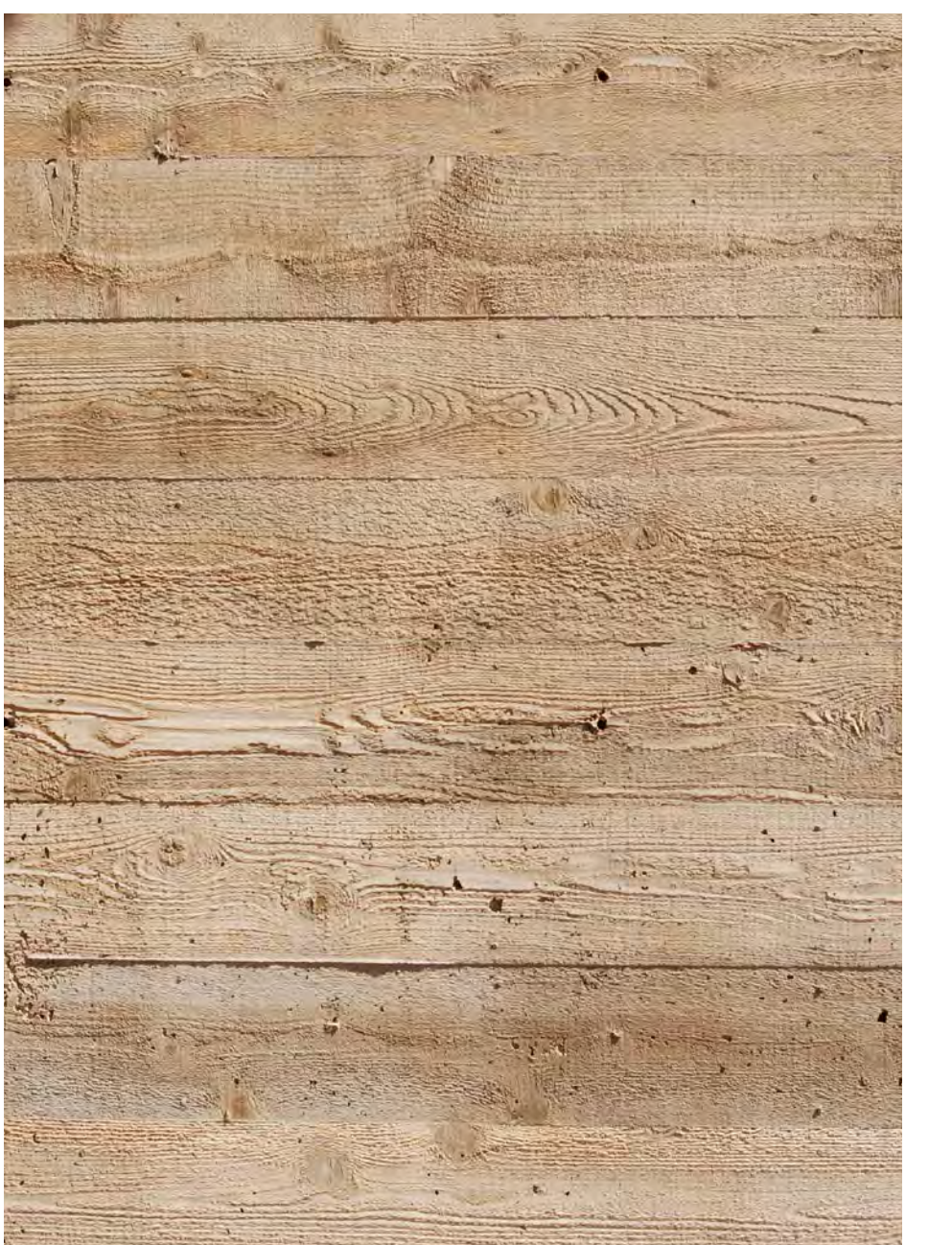
BOARD-FORMED CONCRETE - cast-in-place and stained.
