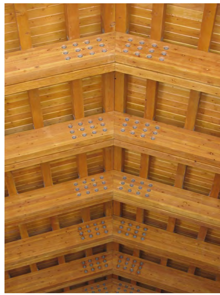
HEAVY TIMBER GLULAM BEAMS, RAFTERS AND COLUMNS with painted galvanized structural steel knife-plate connections. Fasteners to be recessed galvanized steel or stainless steel. Clear heart Western Red Cedar heavy timber purlins and T&G decking with resawn finish. Wood clear coat stain.
