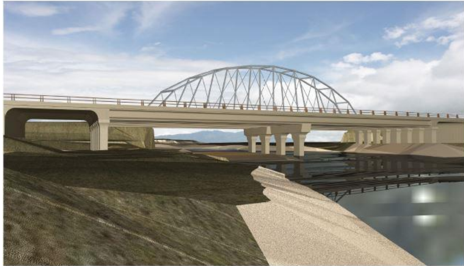
Preliminary Bridge Design Concrete Girder (Looking West from South Bank) 230-ft Long, 2-Span Bridge with “Jump Spans” at ends
