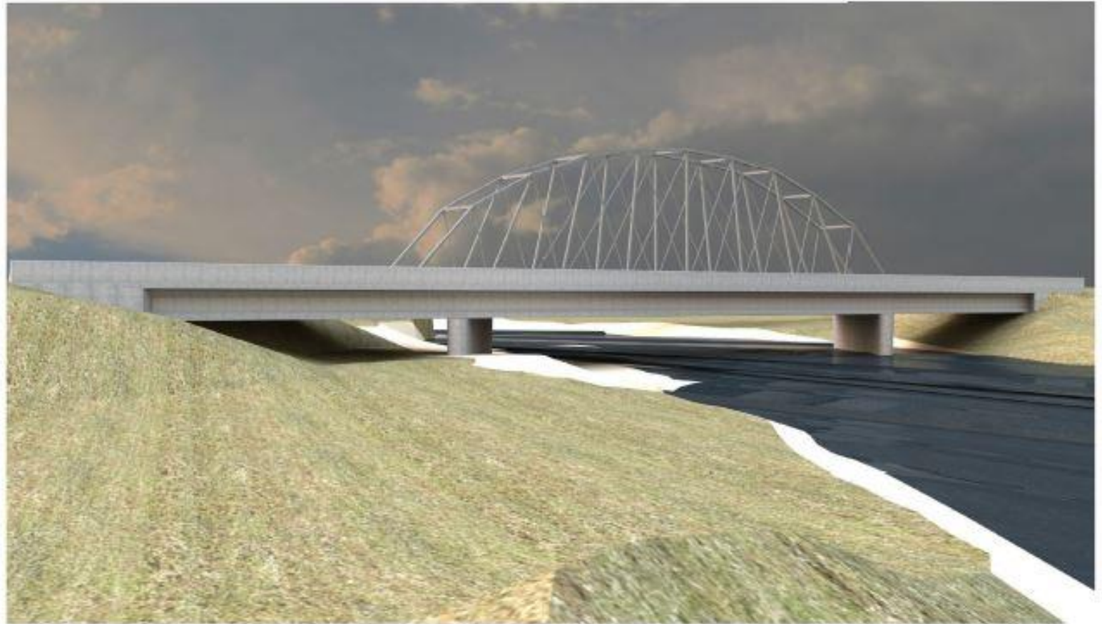
Existing SH-75 Bridge (Looking West from South Bank)
