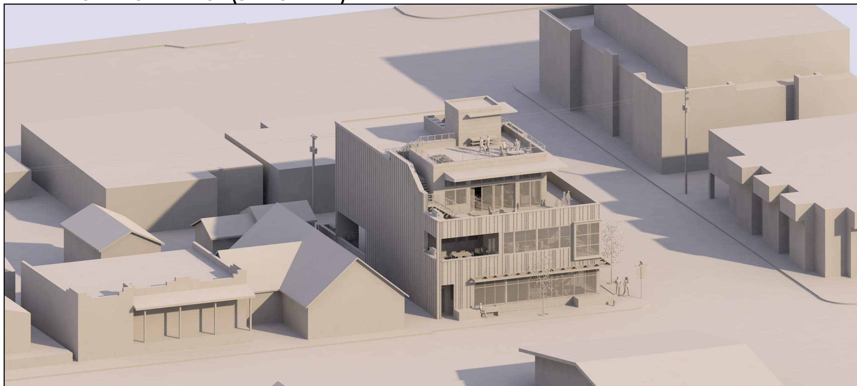
CONTEXT VIEW FROM SOUTHWEST
