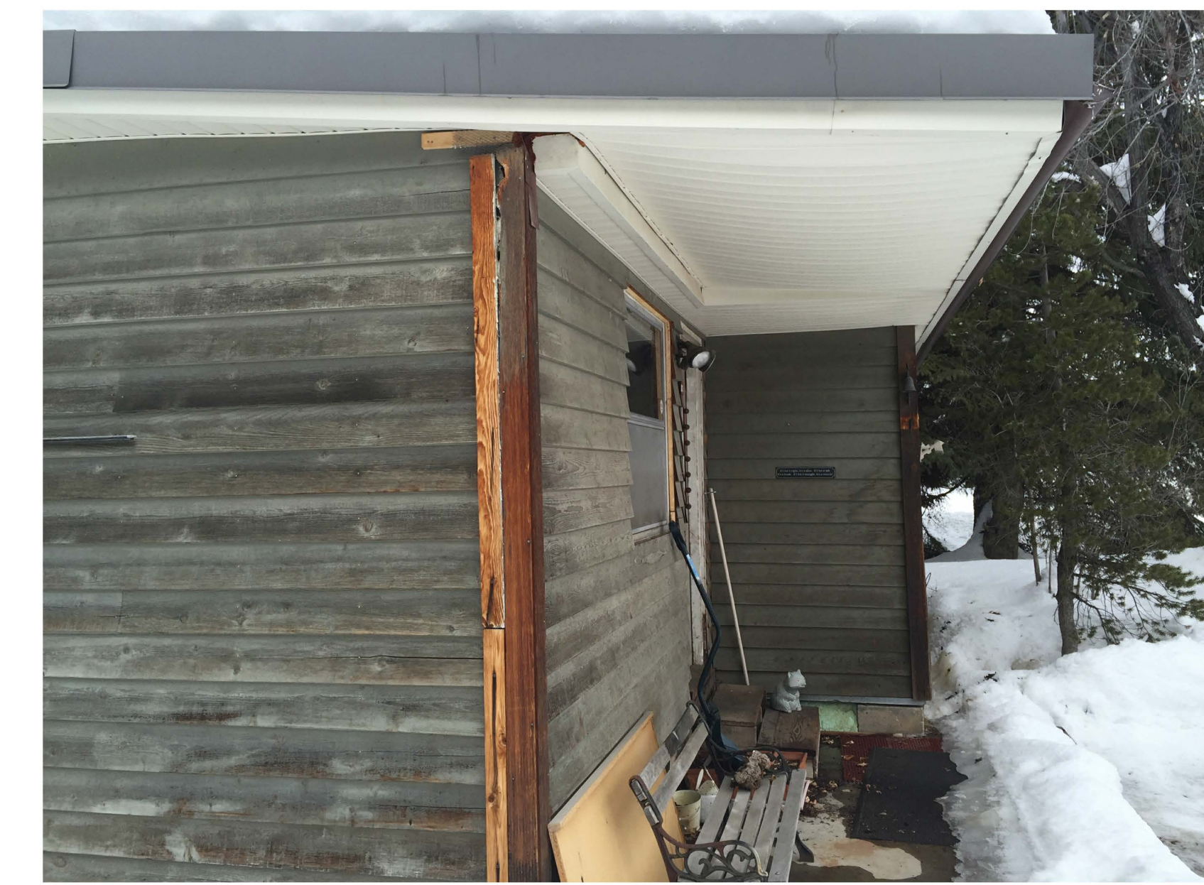
EXISTING STRUCTURE TO BE REMOVED
