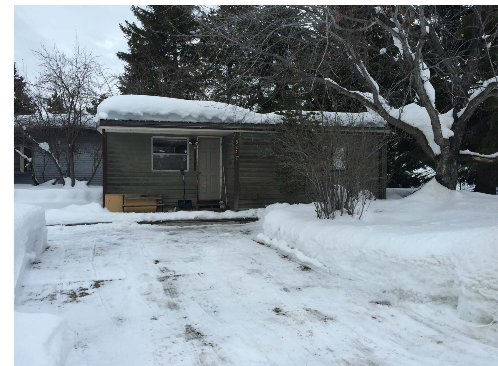
EXISTING STRUCTURE TO BE REMOVED
