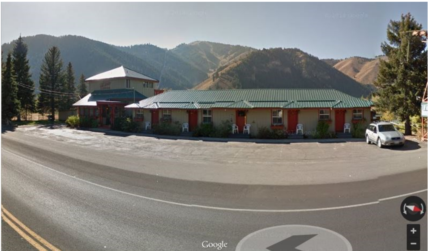
Street View of Lift Tower Lodge 2
