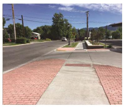
Figure 3: Stamped/colored pavement with rolled curb
