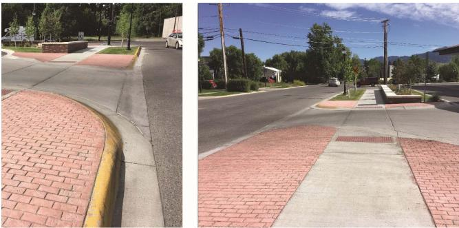
Figure 3: Stamped/colored pavement with rolled curb
