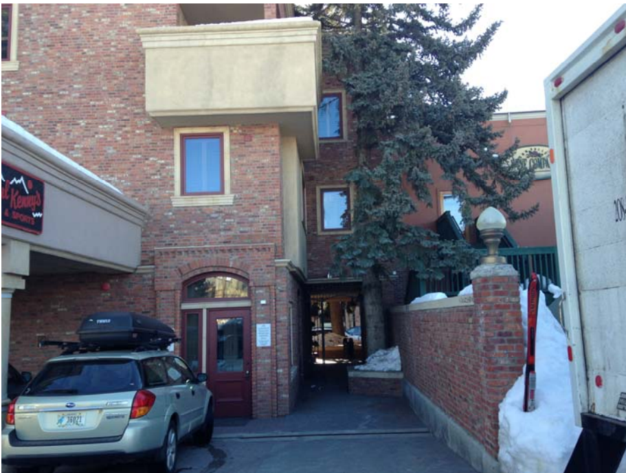
NORTH END OF EAST ELEVATION
