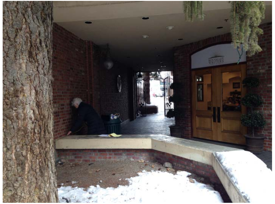
EXTERIOR LIGHTS @ PROPOSED ADDITION
