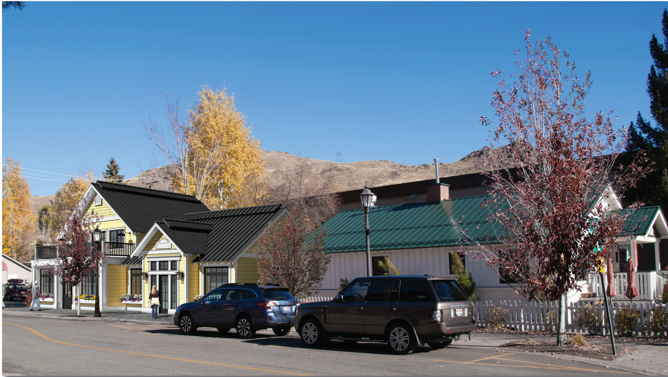
NORTH WEST ELEVATION AS VIEWED FROM FOURTH STREET
